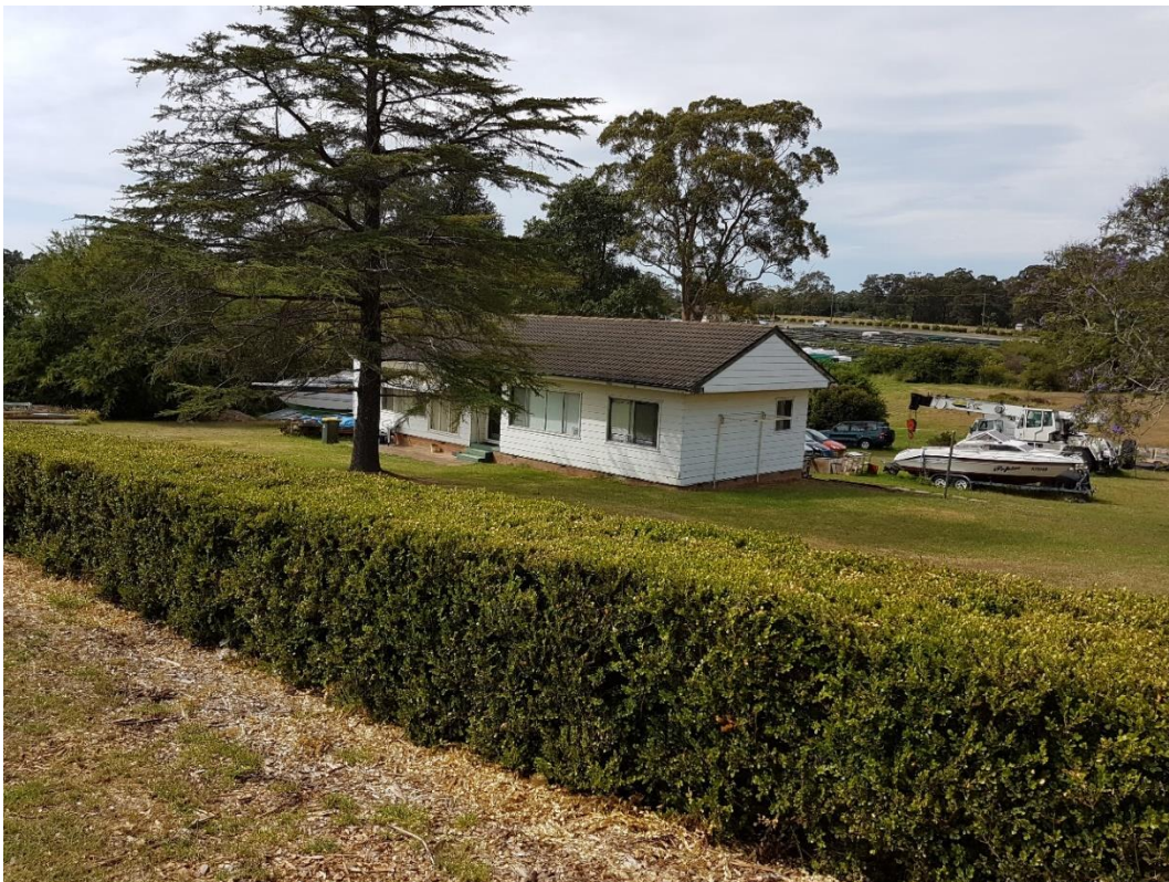
Image 6: The northern site boundary has an existing single storey brick house and green areas
