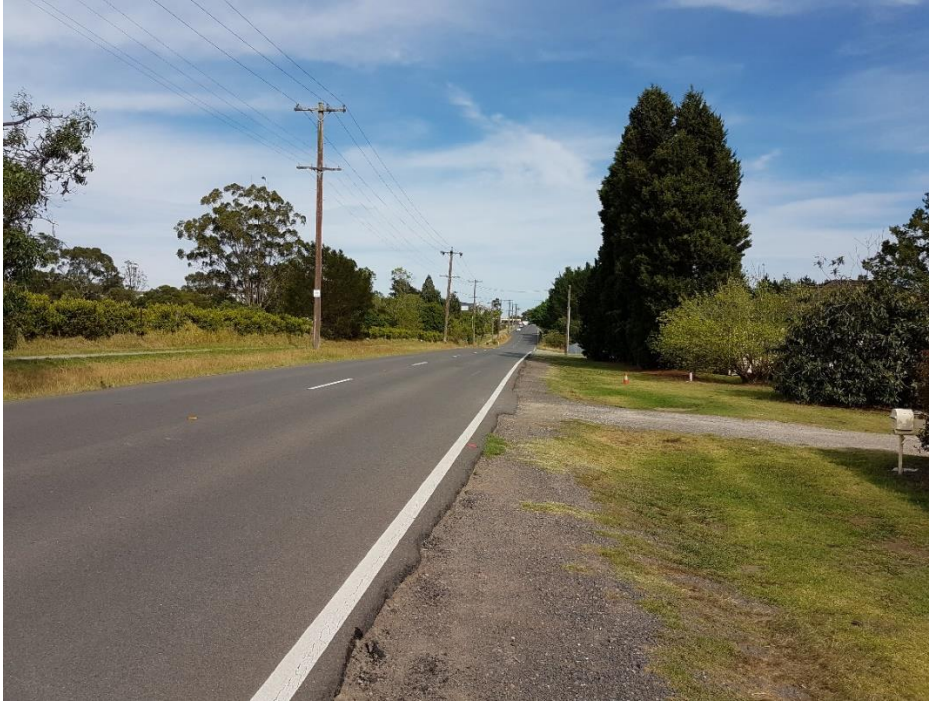
Image 1: Quarry Road has a road fall towards east
